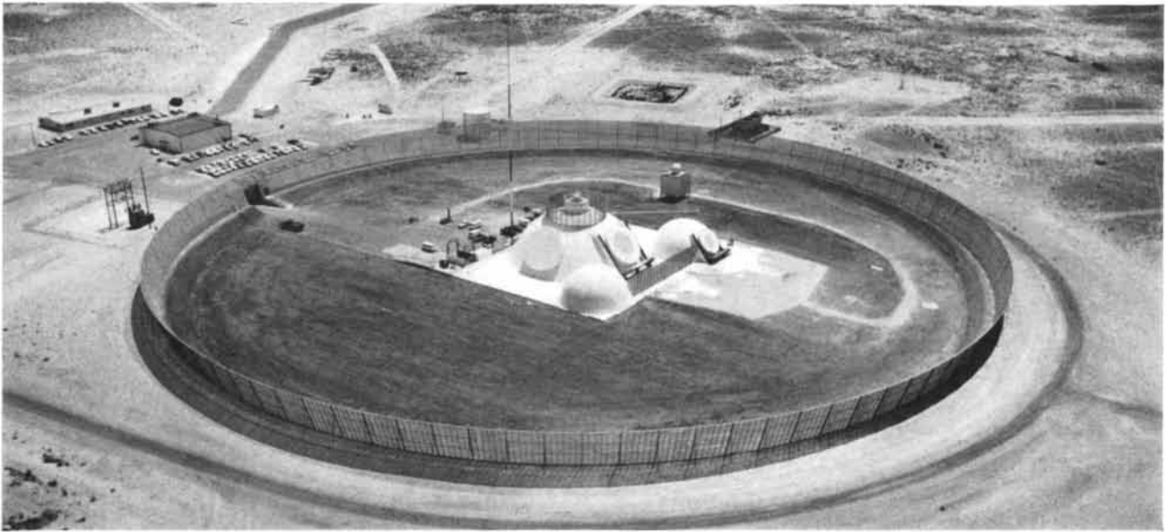
PROTOTYPE OF MISSILE-SITE RADAR is the multifunction array radar (MAR) at the Army's White Sands Missile Range in New Mexico. MSR, a smaller version of MAR, will be used
